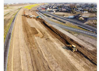
Levee protection works
